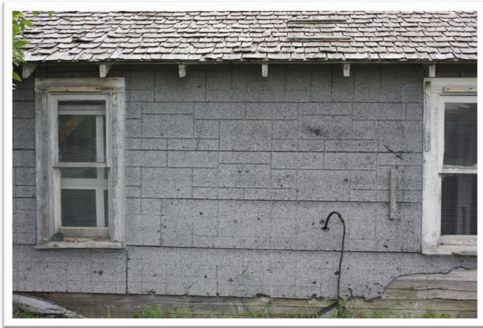
Photo 3: Example of embossed rolled roofing, used as siding
